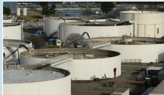
Water and Wastewater Treatment
